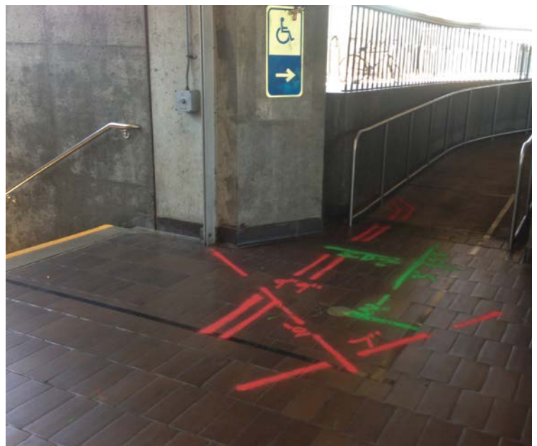
The results of the scanning and imaging work will assist in the installation of strengthening devices on buildings and structures.
