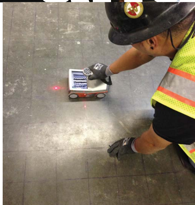
Operators performed GPR imaging in station buildings and outdoor parking areas.
