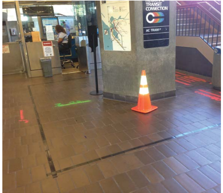
This form of non-destructive testing enabled station operations to continue as usual.
