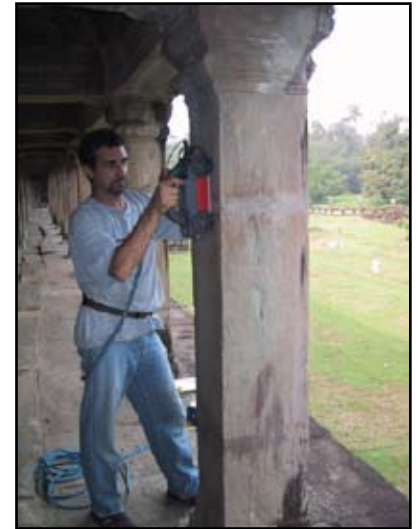
Figure 1 . GPR scanning at "small" column at east column line. The metal ties are evident at the radar trace (below) as is the signal attenuation near the base of the column.
